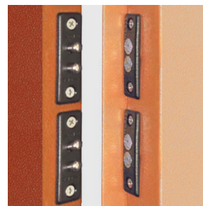
Double electrical contacts between leaf and doorframe
